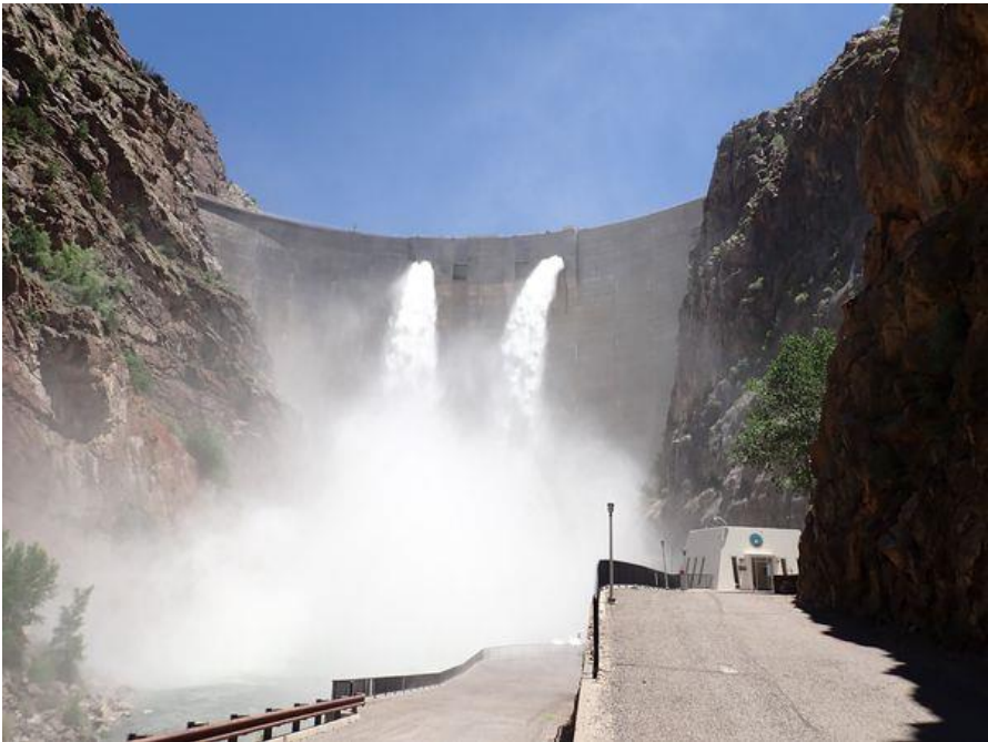
FIGURE 10. Blue Mesa Dam using the spillway in the spring 2023 due to snowmelt.
