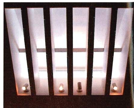
CLERESTORY WINDOWS, OR SUNSCOOPS, PROVIDE NATURAL LIGHT WITH NO ELECTRICITY DURING THE DAY.
