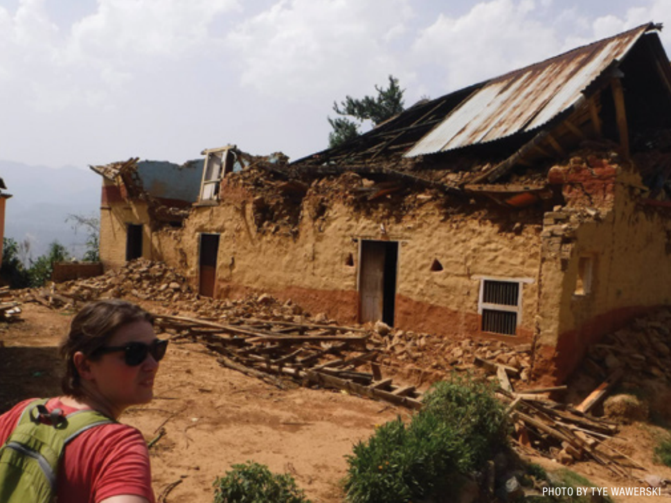
ABOVE: Cain views some of the hundreds of buildings in rural Nepal that were damaged or destroyed by the 7.9 earthquake and its aftershocks.
