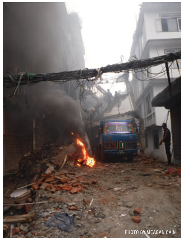
BELOW: Three months after the April 25 earthquake, a section of Kathmandu’s shopping district usually clogged with tourists is still a disaster zone, with residents burning insulation off electrical wire salvaged from destroyed buildings.
