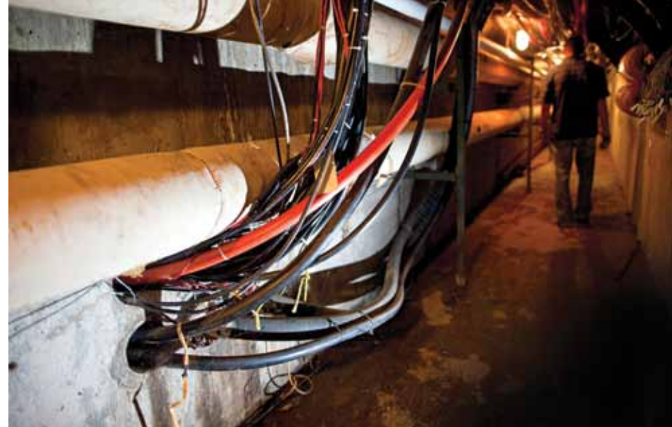
FROM GRAY TO GUNTER: Neighboring Gray Hall is the system's starting point. The NeoBells are programmed taking advantage of digital technology. From there, a maze of wires heads underground to Gunter and up to the building's tower.
