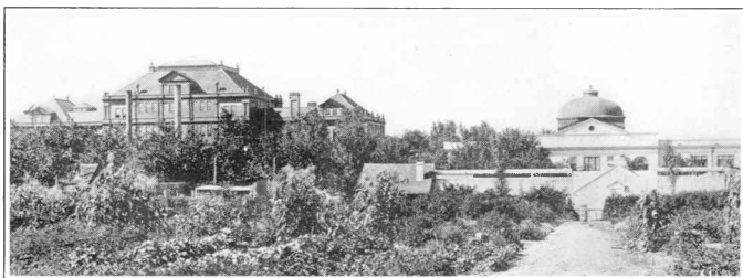
The Buildings from the Rear.
