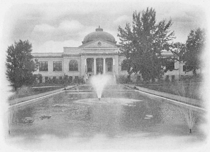
THE LIBRARY, POOL, AND FOUNTAIN.
