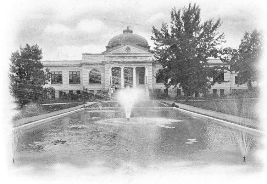
THE LIBRARY, POOL, AND FOUNTAIN.
