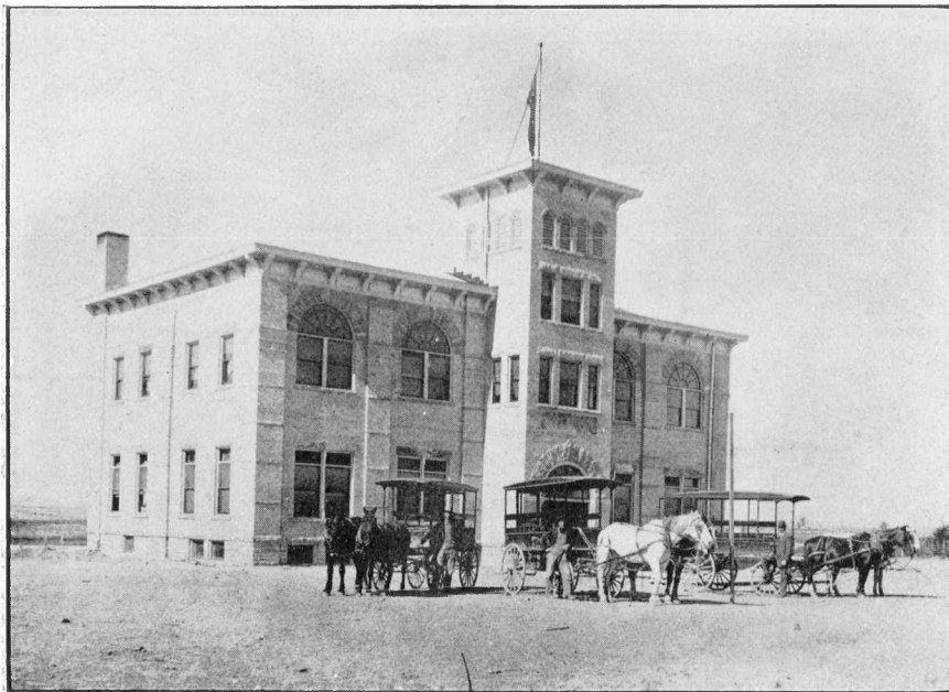
Loma Consolidated School Bilding, Mesa County, Colorado.
