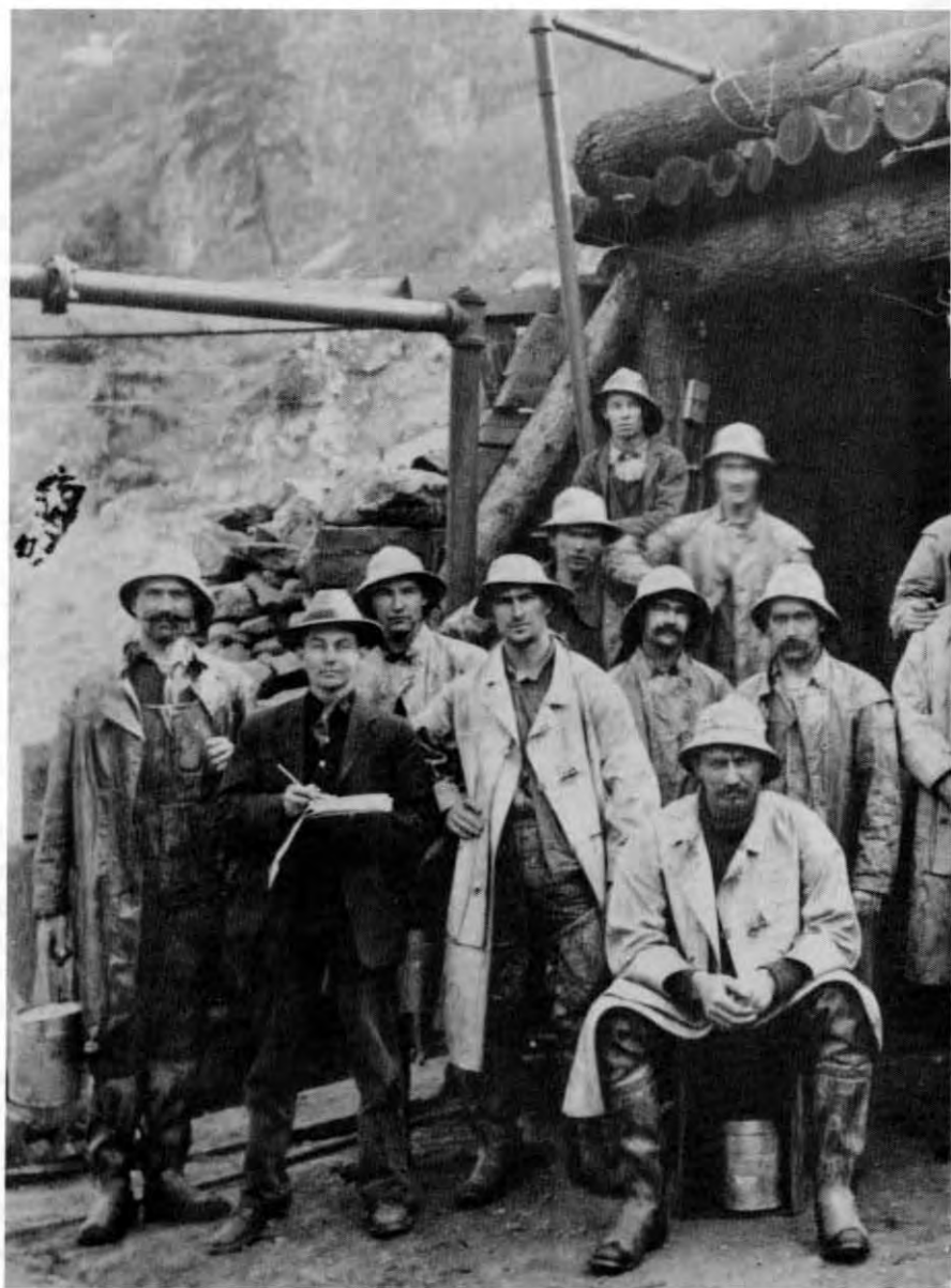
Work crew at the East (River) Portal of the Gunnison Tunnel.
