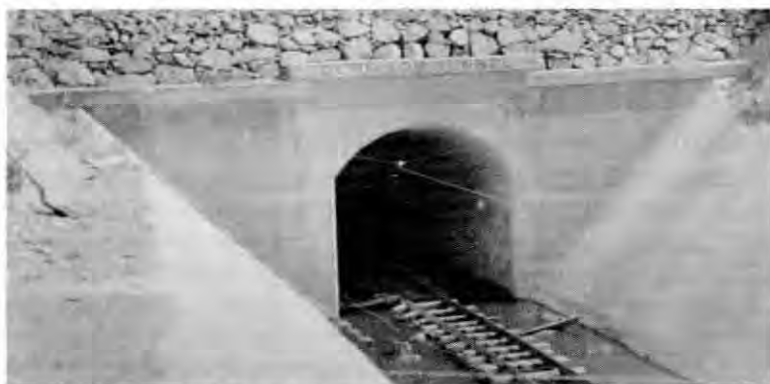
West Portal - Gunnison Tunnel during construction
