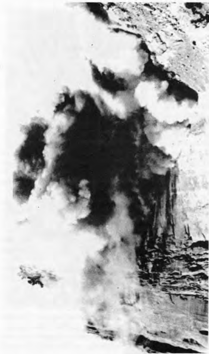
Blasting on highway construction on the Colorado National Monument.
