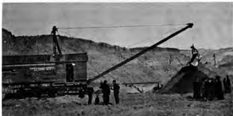
Photo courtesy of The Museum of Western Colorado (Palisade Library Collection 49.23.38) Digging the High Line Canal.
