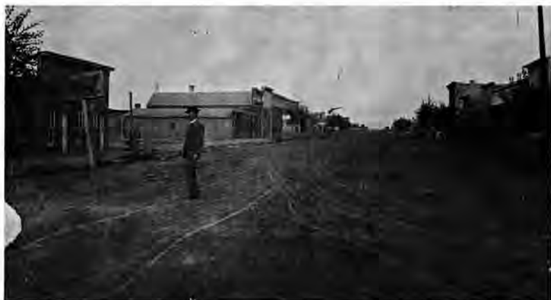
Courtesy of The Museum of Western Colorado (Chamber of Commerce Collection) Looking east, Hoodoo Street, 1880
