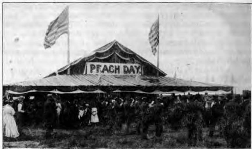
Photo courtesy of Museum of Western Colorado
