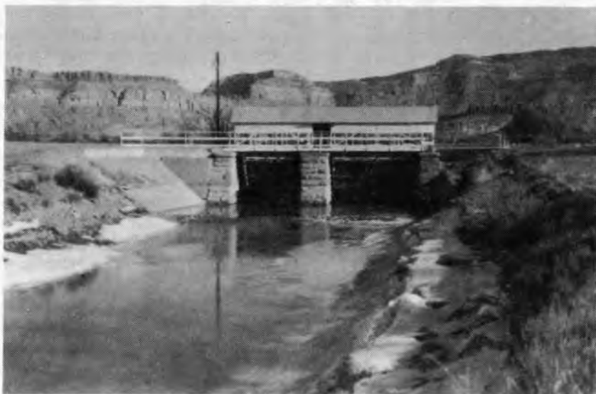
The steel headgates as they are today. After an engineering inspection in 1962, the headgates were declared to be in excellent repair.
