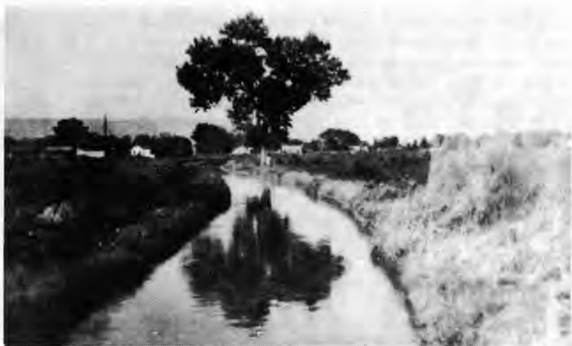
Photo courtesy of the Grand Valley Irrigation Company
