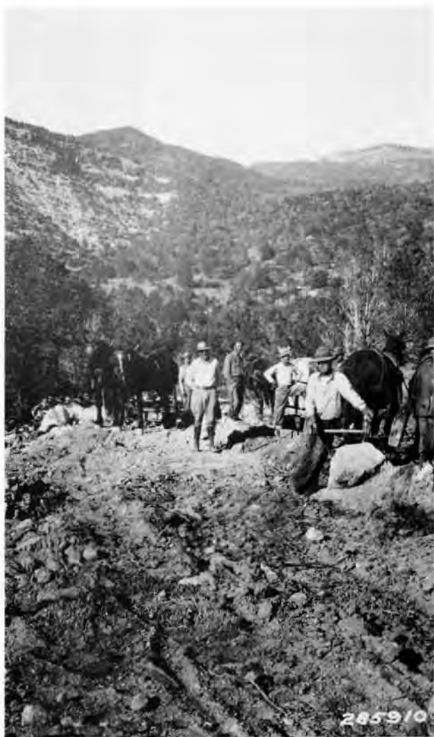
Photo courtesy U.S. Forest Service, Collbran, CO Working on the Lands End Road
