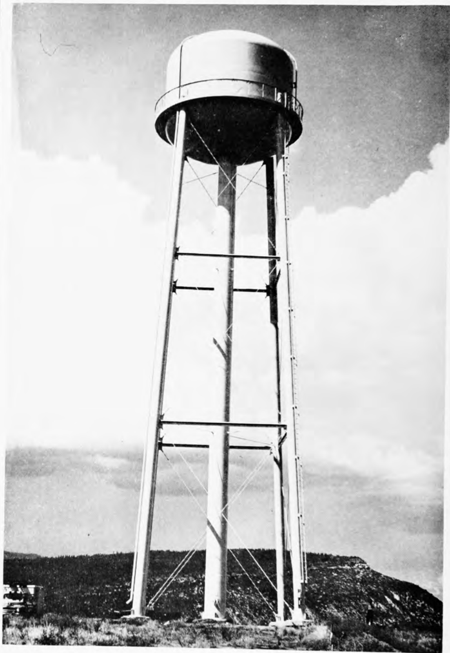
College Water Tower
