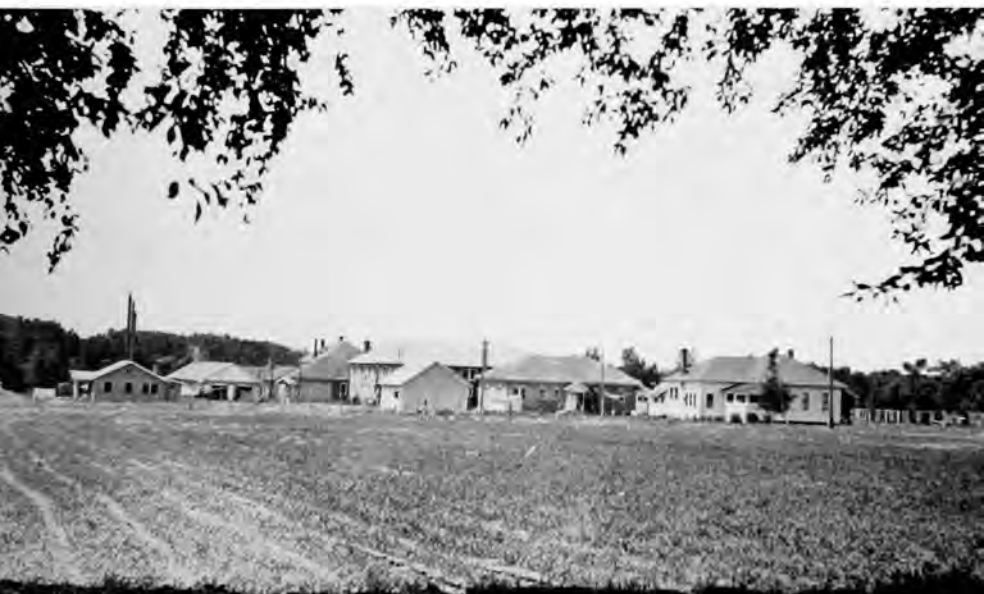
A Number of the Buildings as Seen from the Northeast
