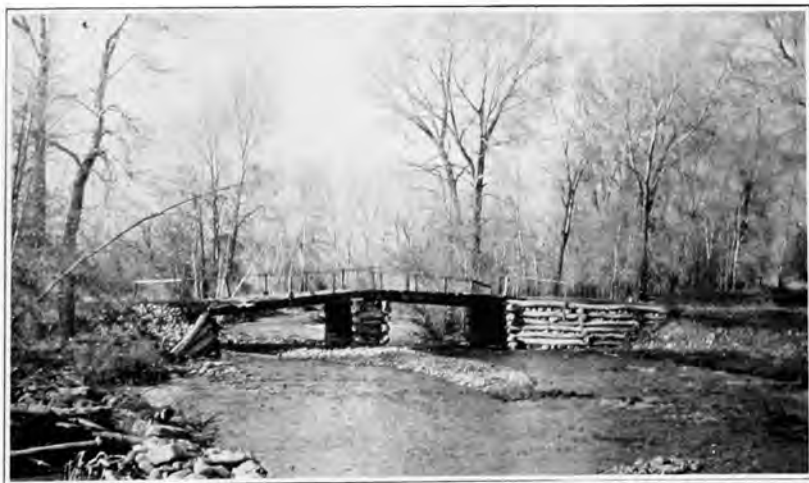
La Plata River Bridge
