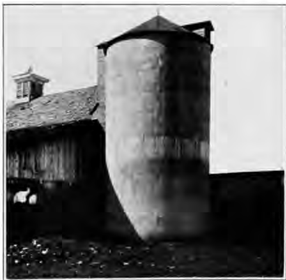
The Concrete Silo, Capacity 100 Tons
