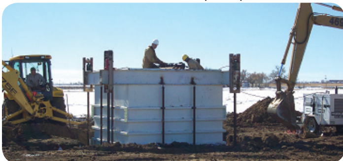
Fig 1: The inner tank being pushed into the ground to acquire the soil monolith. Photo taken by Dale Straw of DWR.
