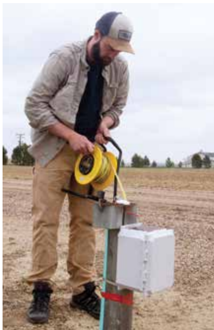
Figure 2. Zach installing a real-time sensor system at CSU's Agricultural Research, Education, and Development Center (ARDEC). Photo by Kelsey Provost.
