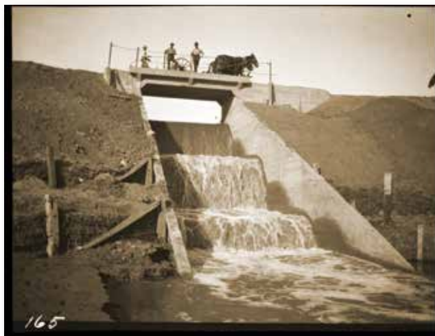
Drop structure in Satanta Canal, c. 1907-08.
