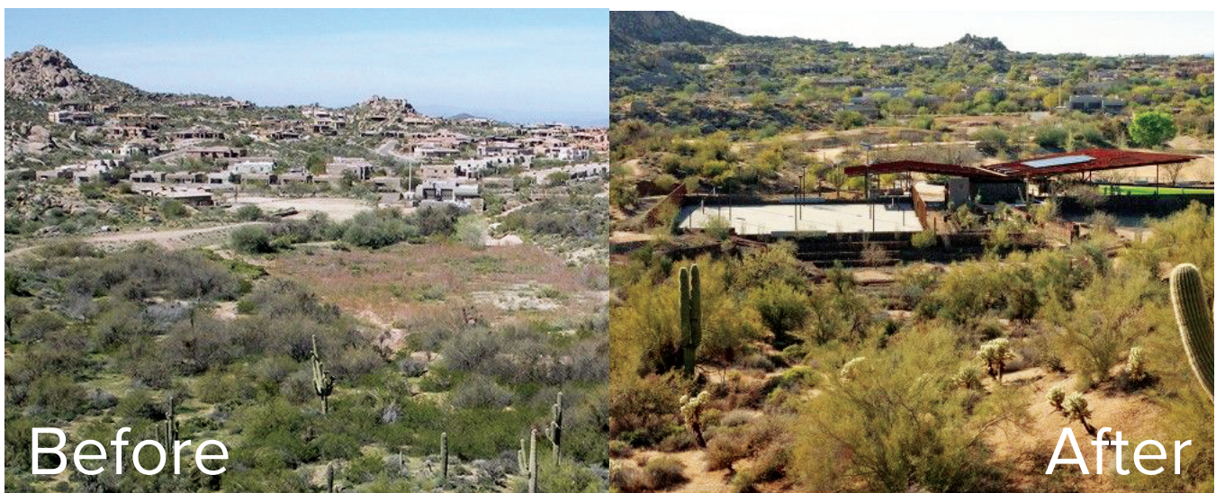
George “Doc” Cavalliere Park, in Scottsdale, Arizona, is a case study project representing beneficial landscape performance metrics with environmental, social, and economic benefits. These images show the site before and after the construction of the park. On the left, a view of the existing basin displays overgrown invasive species, while on the right, the core park elements, basketball courts, restrooms, shaded playground, and turf area are carefully sited in the gabiion lined basins.
