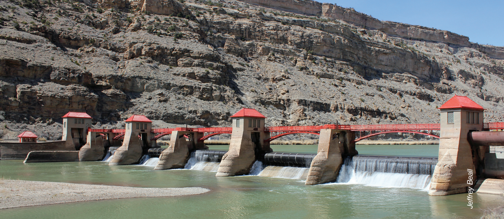
Colorado's famous Grand Valley Project Diversion Dam just east of Grand Junction along I-70. Known as the "Roller Dam" for its multiple cylindrical moving crests, it diverts water into the Government Highline Canal for use by irrigators in Grand Junction. The canal was the site of a large-scale efficiency improvement project completed in 2002.
