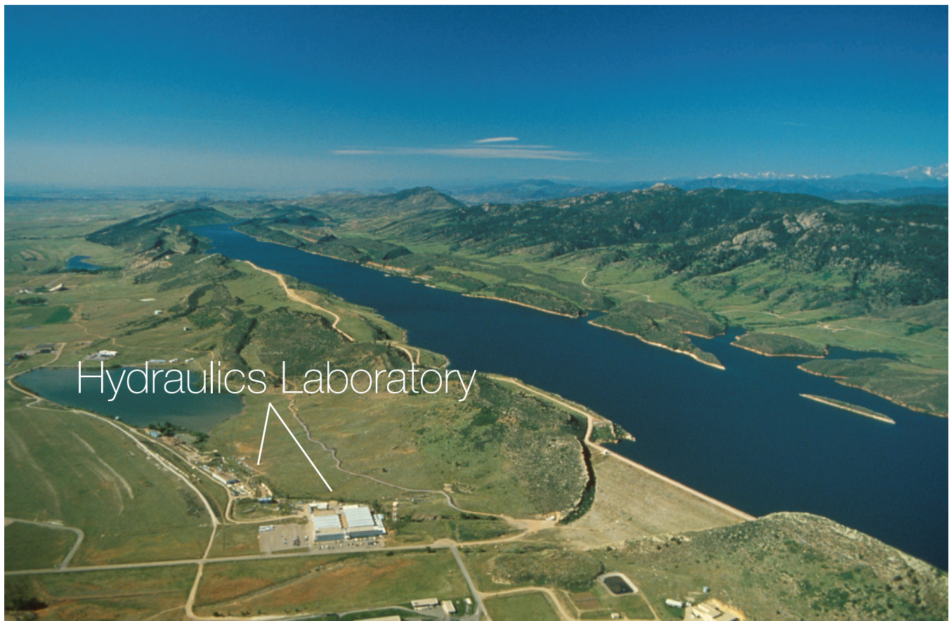
Figure 1. An aerial view of CSU's Hydraulics Laboratory at Horsetooth Reservoir.
