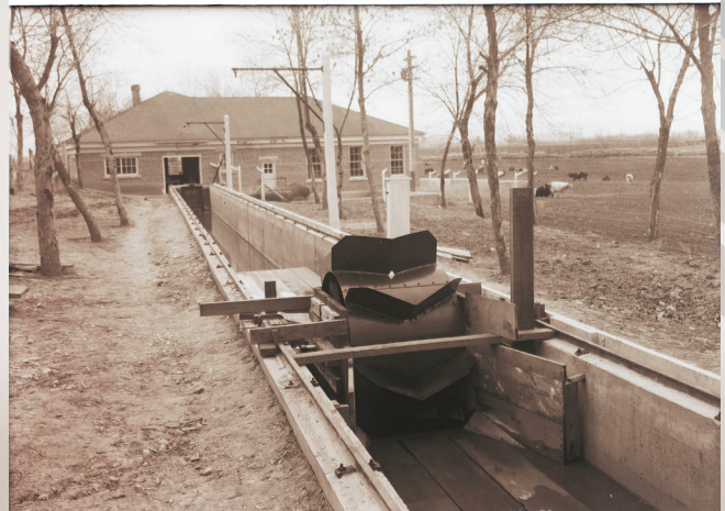
Work at the lab included studies on flumes, weirs, orifices, seepage, sedimentation, evaporation, and various types of meters. The team tested the Dethridge meter, an Australian invention, in the lab's rating tank in 1915.
