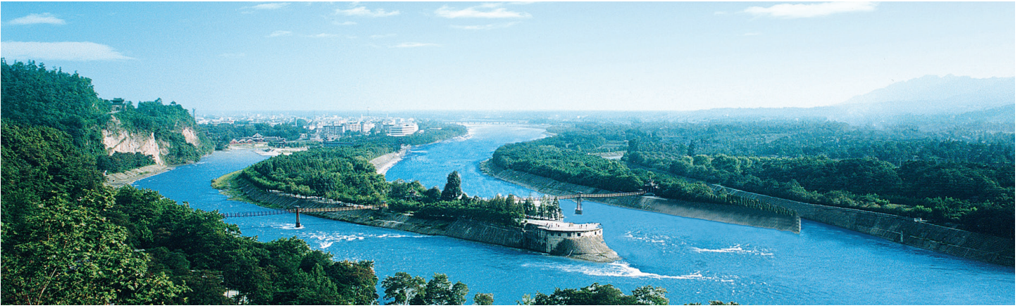
The Yuzui Water-dividing dike is part of the Dujiangyan irrigation system near Chengdu, China. The system dates back more than 2,000 years.
