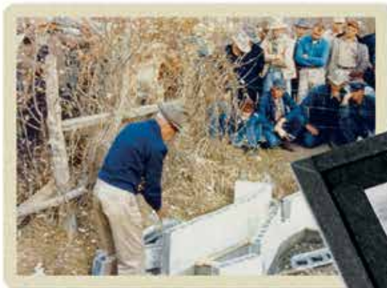
Above: Ralph Parshall conducts a flume demonstration. Right: A lantern slide from the Ralph Parshall archive collection shows constructed flumes. Courtesy of the Water Resources Archive, CSU Libraries
