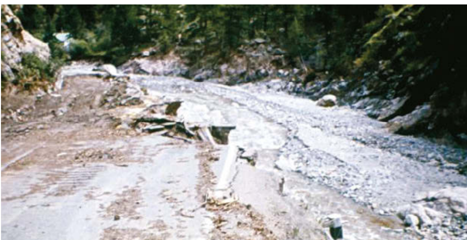
Figure 3. U.S. Highway 34 and the Big Thompson River in the aftermath of the 1976 flood. Note the eroded road where the structure had constricted the canyon watercourse. Courtesy of Maurice L. Albertson Papers, Water Resources Archive, Colorado State University Libraries
