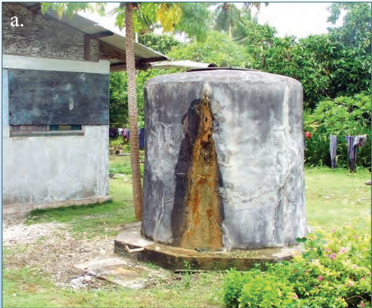
Figure 1. (a) Example of a currently used household rainwater catchment system on Ulithi Atoll that employs a ferro-concrete tank in a state of minor disrepair; (b) shows a rainwater catchment system schematic detailing the various parts of a functioning system, including the roof catchment area, water transmission system, and storage tank.
