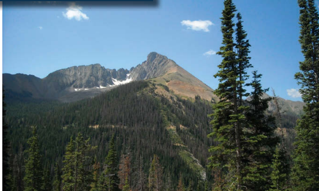
Michigan Ditch (the line in the trees that looks like a road) carries water from Michigan River over Cameron Pass to Joe Wright Reservoir where water then flows into the Poudre River. The ditch redirects the water flow to Fort Collins from its natural route towards Wyoming.
