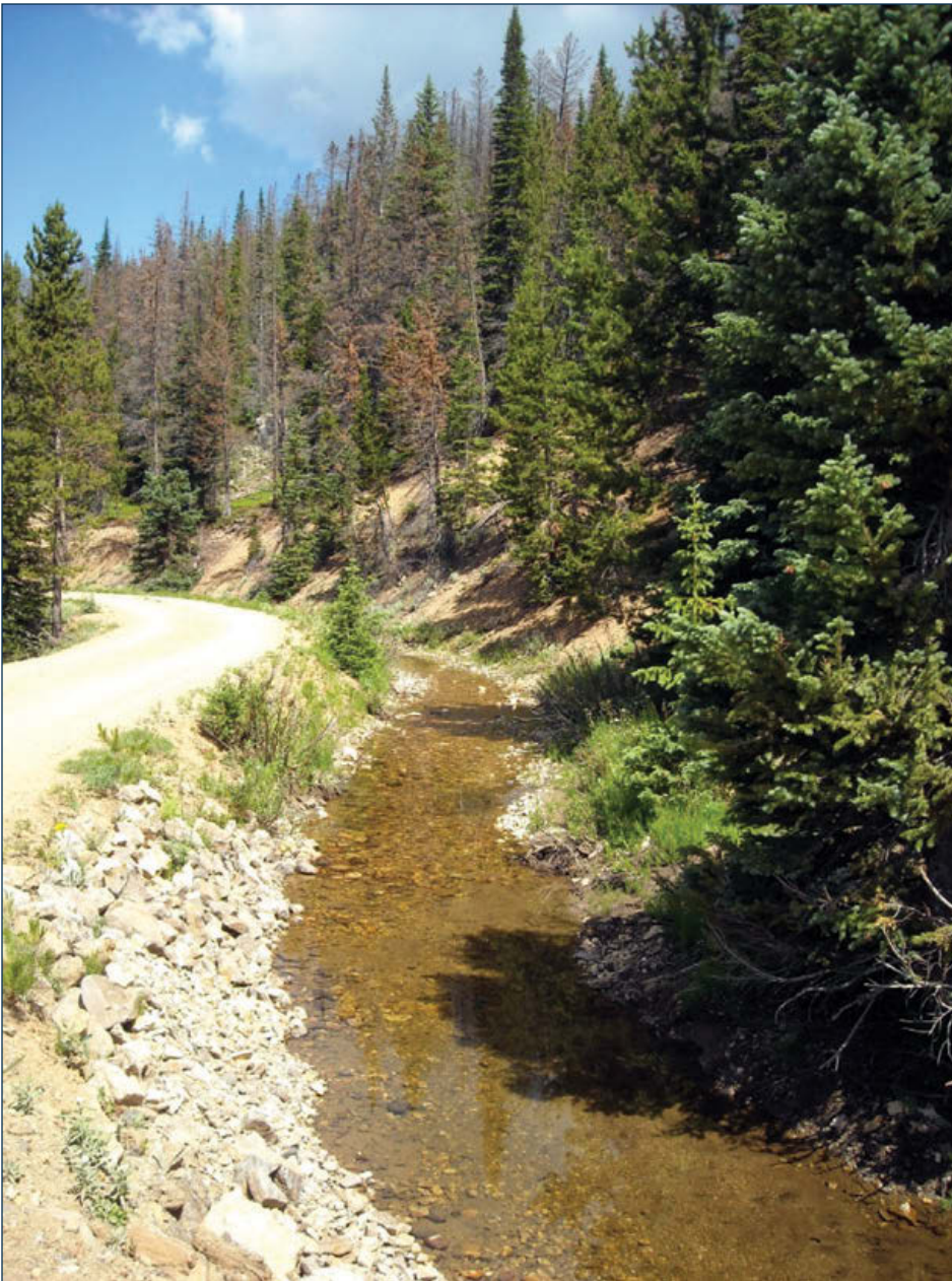
In 1971, the city of Fort Collins acquired Michigan Ditch and Joe Wright Reservoir near Cameron Pass to plan for the city's growing water needs. Constructed in 1902, the ditch and reservoir system required extensive renovations, resulting in one of the largest projects the utilities had undertaken until then. The utilities completed the expansion and renovation in 1980.
