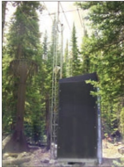
A SnoTel site from Hourglass Reservoir near Pingree Park.
