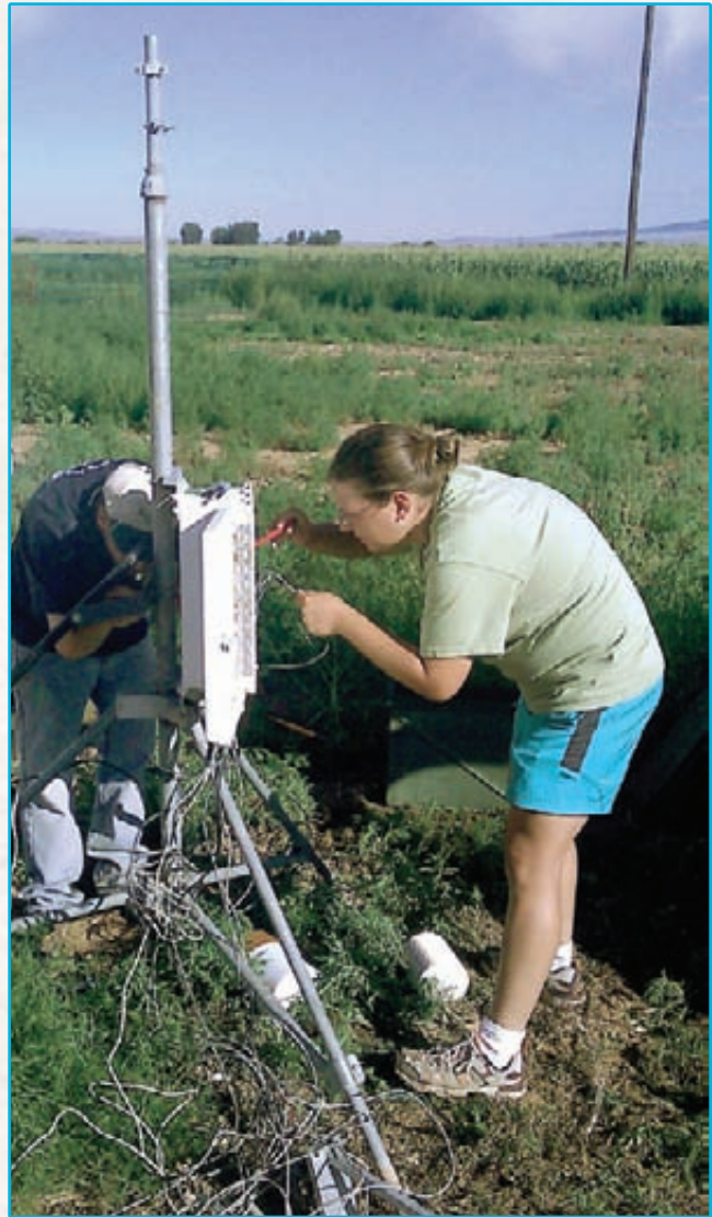
Wendy Ryan and Noah Newman of the Colorado Climate Center install a CoAgMet Weather Station.
