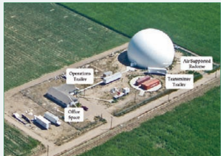
Figure 2. The CHILL radar site near Greeley, Colo., as seen from the air.
