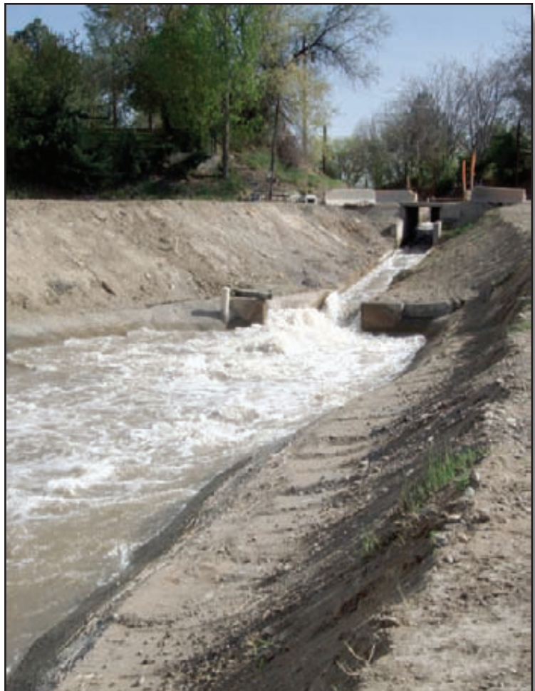
This ditch is a good example of a Colorado irrigation canal with "micro-hydro" (small-scale hydropower) potential.
