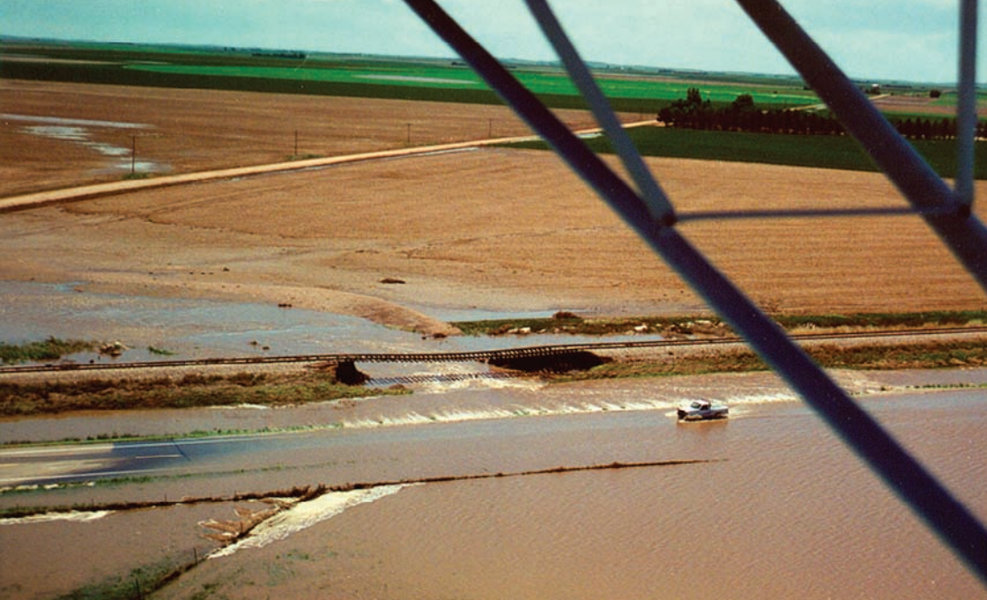
The 1997 flood on Pawnee Creek in Colorado washed out the Holyoke Railroad bridge.
