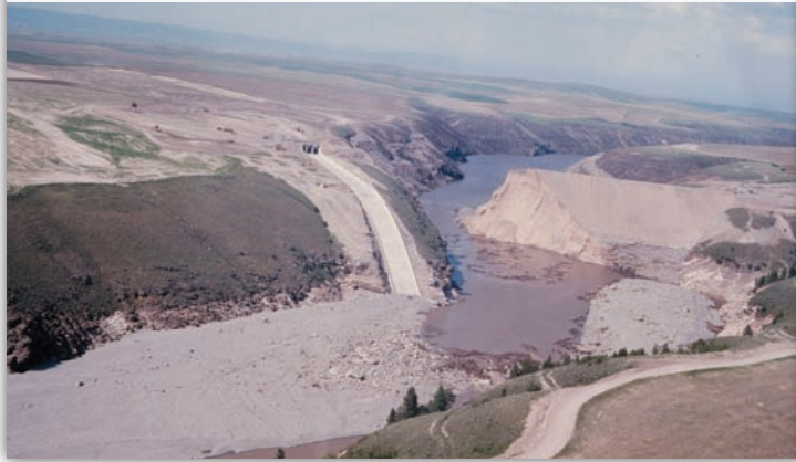
This image shows the Teton Dam on June 6, 1976, after its failure. (Image from Stamm Papers, Water Resources Archive, CSU)
