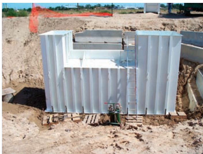
Figure 1. This image shows the retainer tank of the reference lysimeter after being set on the foundation. (Image courtesy of Lane Simmons)
