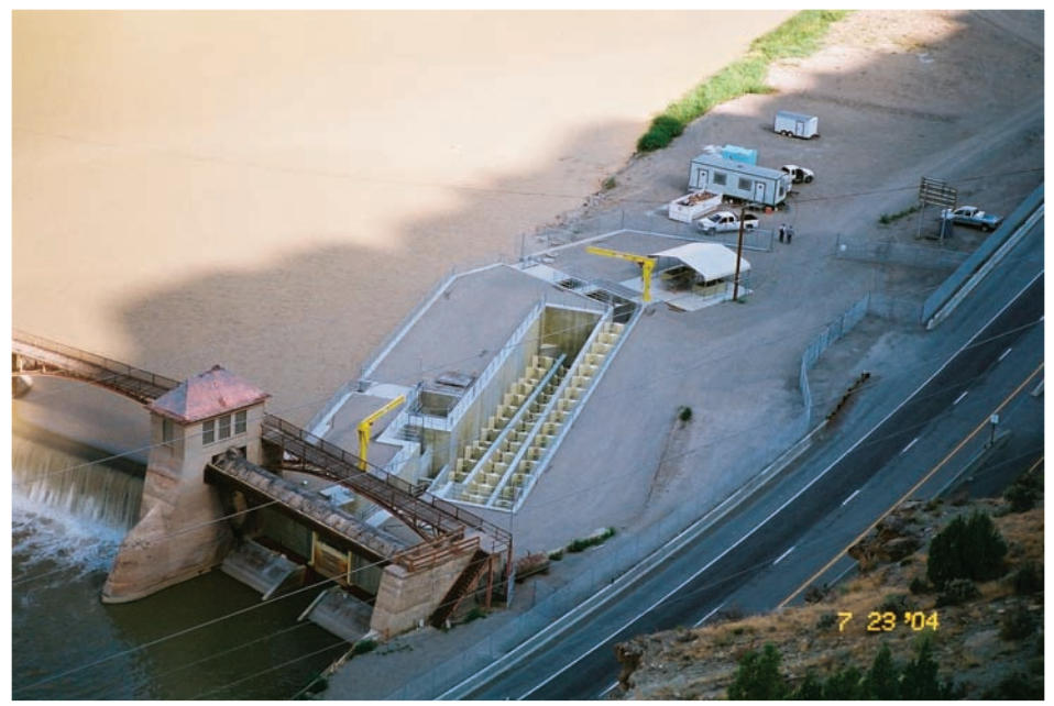
The fish passage at the Roller Dam constructed by the Recovery Program helps provide endangered fish access to 340 miles of critical habitat on the Gunnison and Colorado Rivers. (Image courtesy of Upper Colorado River Endangered Fish Recovery Program)
