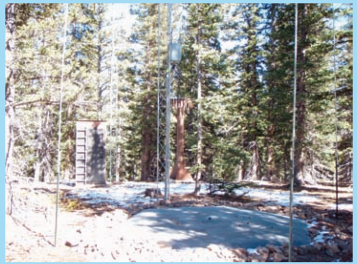
Figure 4. This SNOTEL site was recently installed at Sargents Mesa in the Rio Grande Basin, Colorado.
