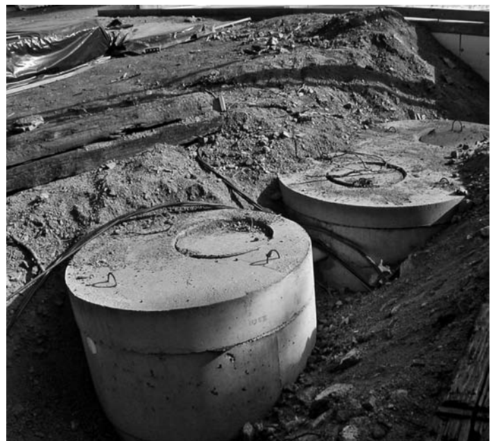
Two-stage septic tank.
