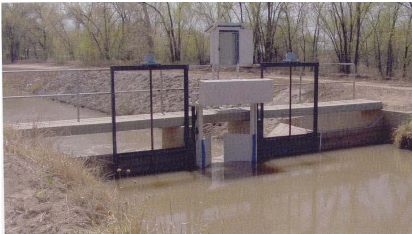
The Lopac gate controls water surface elevation upstream, serving as an automated check structure.
