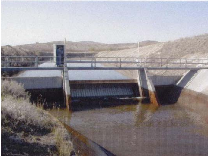
Langemann gates have the capability to maintain constant upstream water level or a pre-determined constant flow rate to downstream users.
