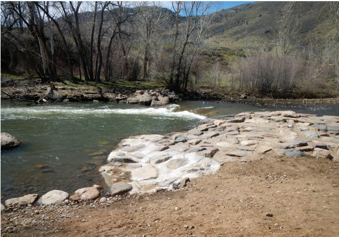
Depiction of shallow depth and high velocities over a grouted chute on Clear Creek in Golden. Courtesy of Tim Stephens
