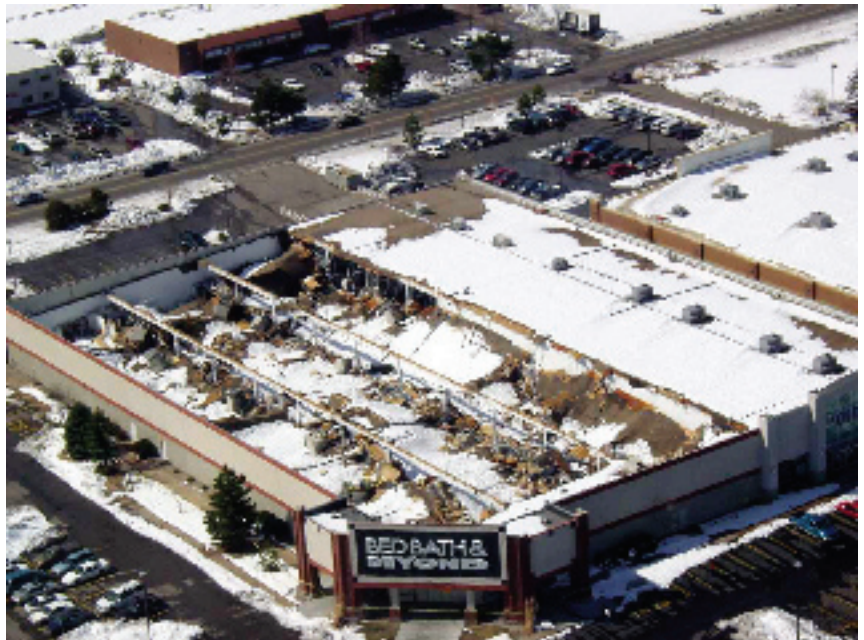
Figure 11. Collapsed roof of the large Bed, Bath, and Beyond store on south College Avenue in Fort Collins, CO. The roof on this structure was replaced and the store reopened several months later. Photo courtesy of Ron Phillips, City of Fort Collins.
