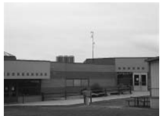
Rooftop Weather Station at an Elementary School in Highlands Ranch, Colo.
