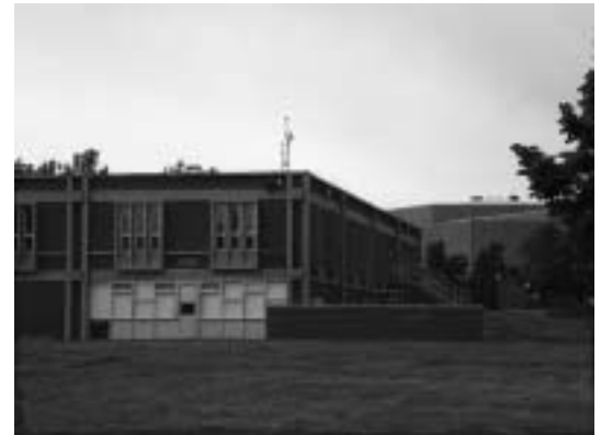
Rooftop weather station at a Middle School in Boulder, Colo.
