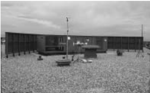
Peakview Elementary School rooftop weather station looking west. Note the proximity to air-conditioning unit. Windbreaks, like this one behind the AC unit, are also present to the north and south (Peak-A site located next to automated site).
