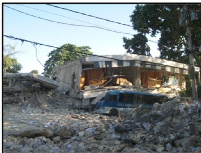
Picture 1. Buildings collapse on a bus in Port-au-Prince, destroying homes and infrastructure.
