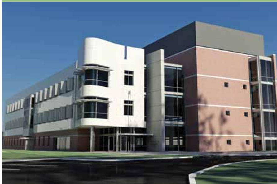
Diagnostic Medicine Center – A 90,000 square foot analytical and diagnostic lab. Paid for by the State of Colorado. Construction started in fall 2007.
