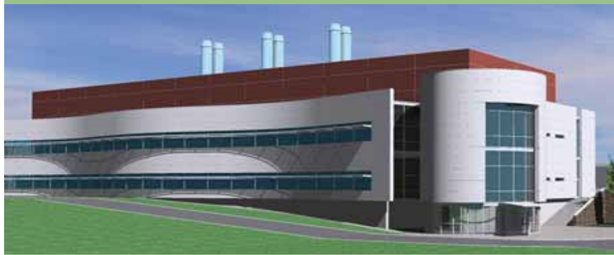
Research Innovation Center (RIC) – Located at the Foothills Campus in the Judson Harper Research Complex next to the Regional Biocontainment Lab. The RIC will be a 60,000 square foot building, cost $52 million, and is scheduled for completion in spring 2010.
