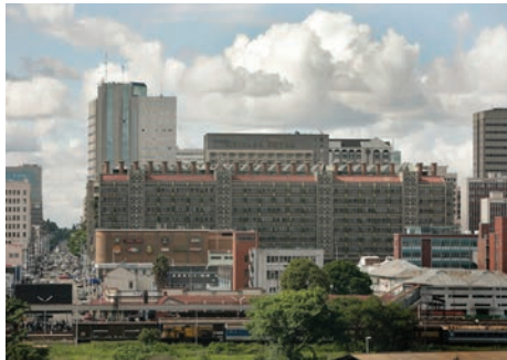
Figure 2. Harare, Zimbabwe: Eastgate Centre with its rooftop chimneys, which serve to drive the passive HVAC system 35 Photo by: David Brazier
