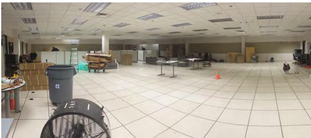
Figure 3. Complete tear down of OPS floor.
