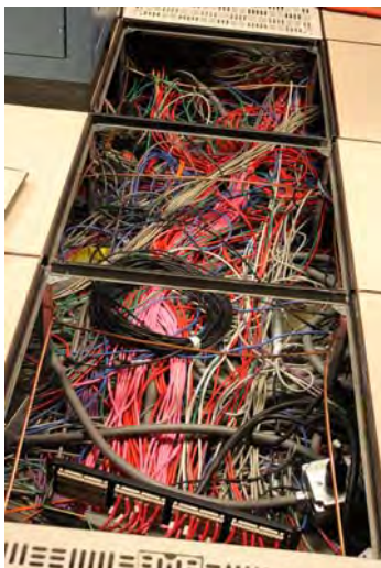
Figure 1. Before cable re-organization.
