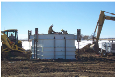
Figure 1. The inner tank of the crop lysimeter being pushed into the ground to acquire the soil monolith. Photo taken by Dale Straw of DWR.
