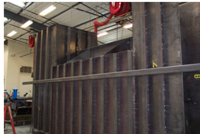
Figure 6. The outer tank and instrument chamber of the reference lysimeter under construction at the USDA-ARS workshop in Fort Collins, CO. On the left side is the outer tank that will hold the inner tank and soil monolith. The midsection will house the weighing mechanism and data loggers, and on the right side is the access hatch. Photo taken by Dale Straw of DWR.
