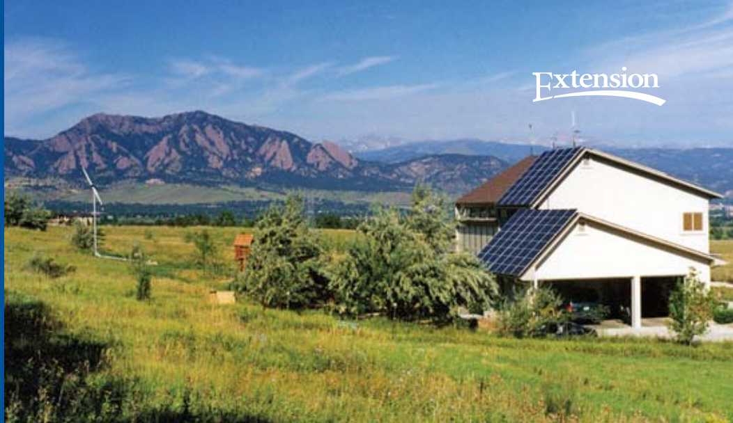
A home in rural Boulder County features a Whisper 3000 (small) wind turbine, passive solar design, and a PV power system on the roof. The wind turbine is rated at 3 kW, has a 14.7 foot (4.5 meter) diameter rotor, and charges a 54 volt DC battery bank. The PV system consists of BP Solar model 590 modules, rated at 8.6 kW. The home also has a pair of Trace SW5548 inverters, 240 volt AC, rated at 11 kW. The home is all-electric, including an electric dryer, stove, oven, and a charger for an electric car. Space heating and cooling are accomplished through a ground-source heat pump.
