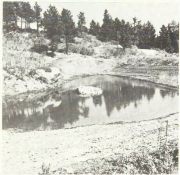
Photo 7--Bentonite has been used for sealing small ponds or reservoirs. It is spread in a layer 1/2 to 2-inches thick over the pond area, worked into the sub-soil, and compacted, if possible.
